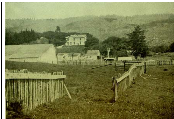
Figure 9-40. This historic photograph of an offset fence near Bolinas, California was taken by G.K. Gilbert shortly after the 1906 earthquake. The offset fence shows a right-lateral slip of about 8.5 feet. Also note the high degree of deforestation shown on the distant hillsides in this photograph. The view of the fence is toward the east.
