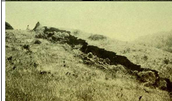
Figure 9-5. View looking southeast along the fault near Point Reyes Station. Note the woman for scale near the top of the hill to the left of the fault scarp.
