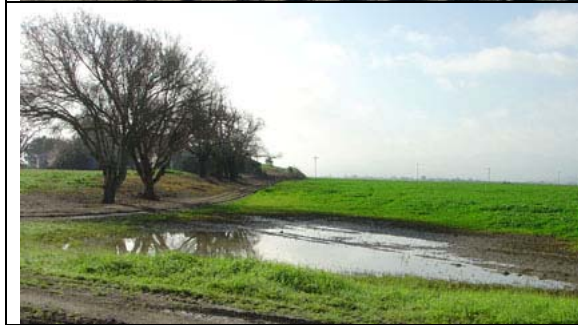
Figure 2-3. A sag pond and low linear scarp along a second strand of the Calaveras Fault on the west side of Highway 25 north of downtown Hollister. This view was taken in the same location as the image above.
