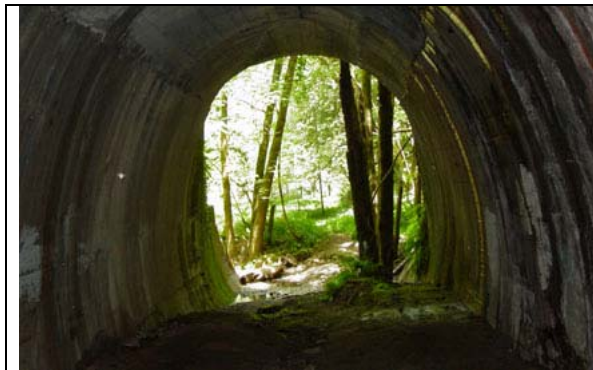
Figure 3-6. View looking out of the west end of Wrights Tunnel toward Los Gatos Creek. The tunnel is now full of leaking cracks that are feeding a small stream flowing from the mouth of the passage.
