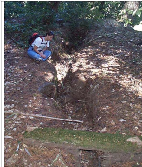
Figure 4-3. One of many fissures along the Big Slide Trail that opened during the 1989 earthquake.
