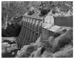
The dam is 124 ft high from foundation to crest and spans 576 ft across the canyon, forming a reservoir with a capacity of 3,700 acre·ft. The reservoir has a surface area of 108 acres and receives water from a drainage area of 63.7 sq mi on the north slope of the San Gabriel Mountains. A formerly popular recreation spot, the dam, reservoir, and vicinity used to receive about 300,000 visitors each year, but since 2015, the facilities have been closed to the public.
